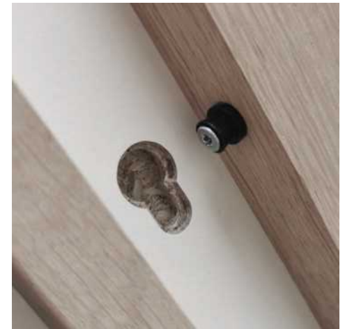
KV pocket for holding solid wood slats
